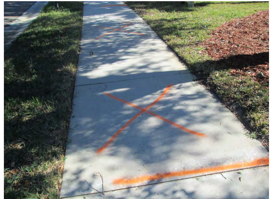
Remove & Replace 2ea of 5' x 5' panels on south Monterey Bay Loop
