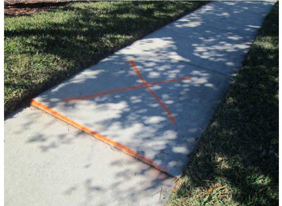
Remove & Replace 5' x 5' on Golden Harbour Tr n/o Kinsbury Place
