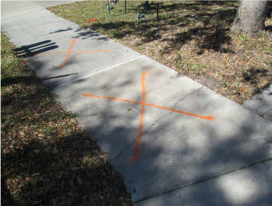
Remove & Replace 13' x 5' on south Chatum Light Run
