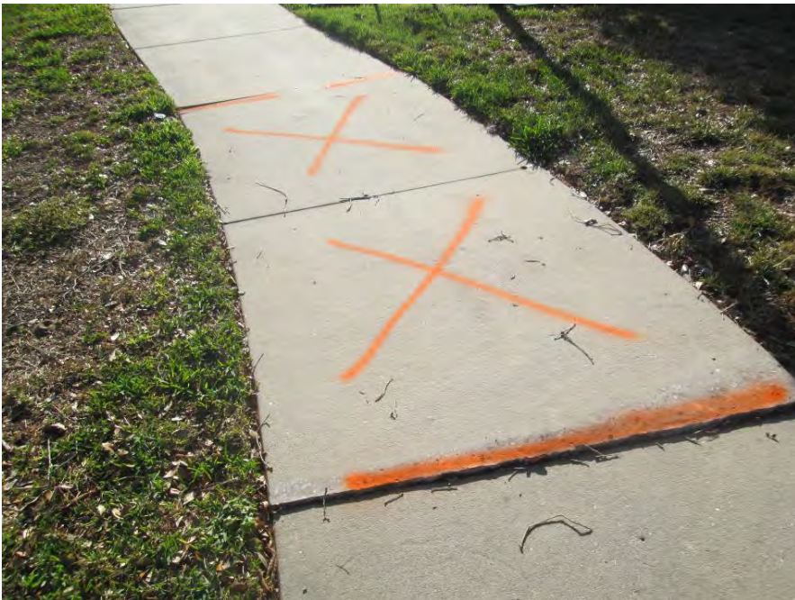
Remove & Replace 10' x 5' at Kinsbury Place cul-de-sac
