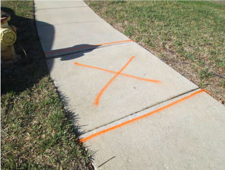
Remove & Replace 6' x 5' on northern side of west Stone Harbour Loop
