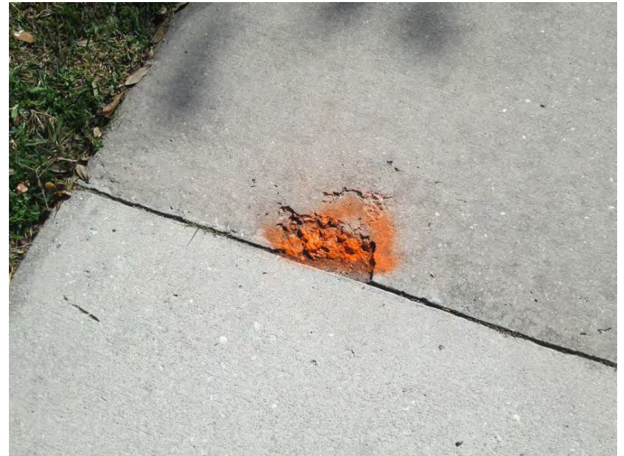
Epoxy grout gouge on Chatum Light Run n/o Beacon Harbour Loop
