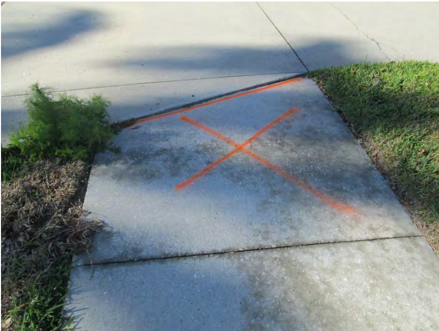
Remove & Replace 4' x 5' on south Stone Harbour Loop
