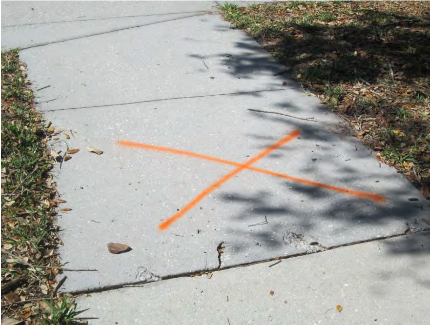
Remove & Replace 5' x 5' on south Beacon Harbour Loop
