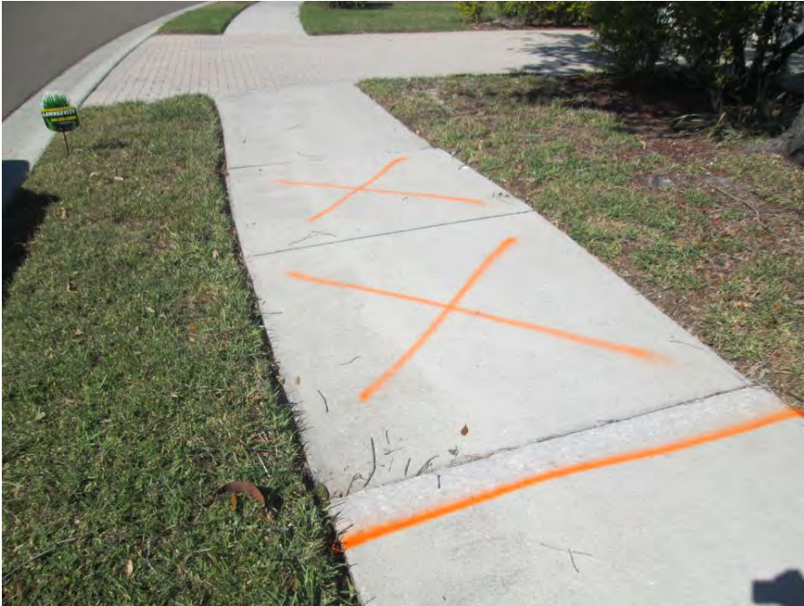
Remove & Replace 10.5' x 5' on Monterey Bay Loop
