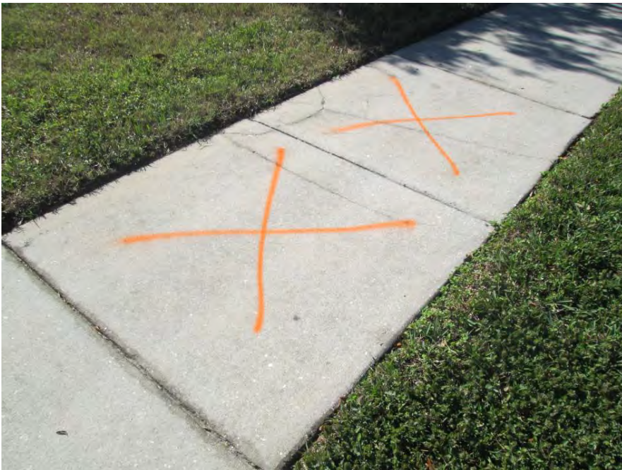
Remove & Replace 10' x 5' on northern west Stone Harbour Loop
