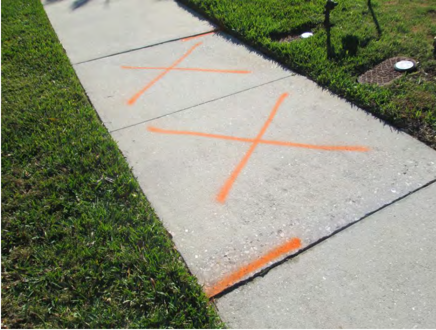
Remove & Replace 10' x 5' on west Stone Harbour Loop
