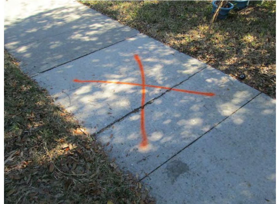
Remove & Replace 5' x 5' on north Chatum Light Run e/o Harbour Lights
