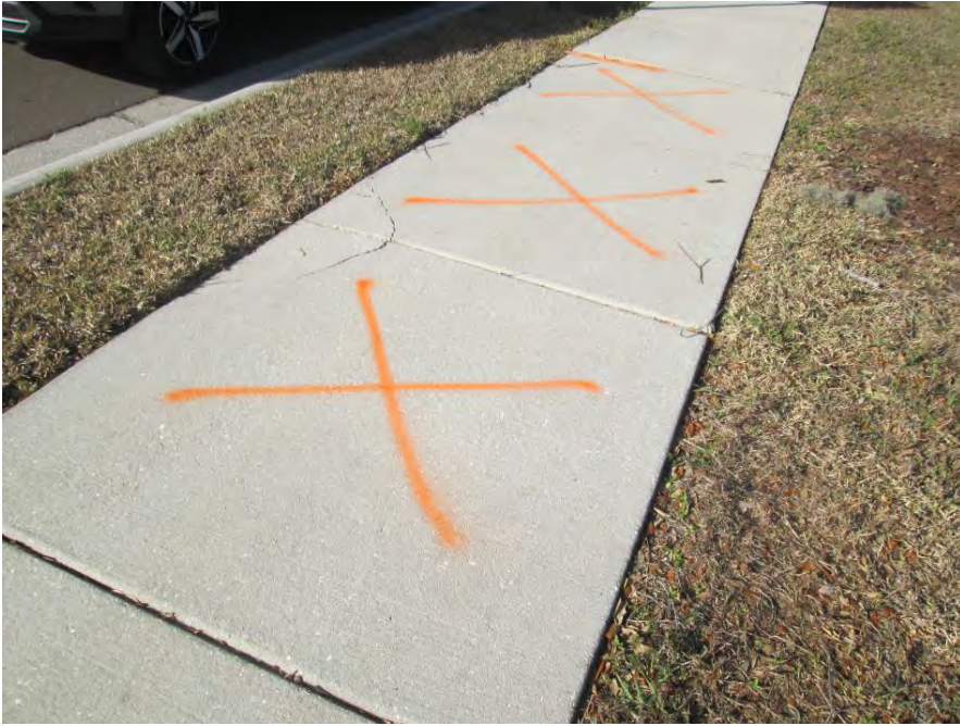
Remove & Replace 15' x 5' on south end of Golden Harbour Dr
