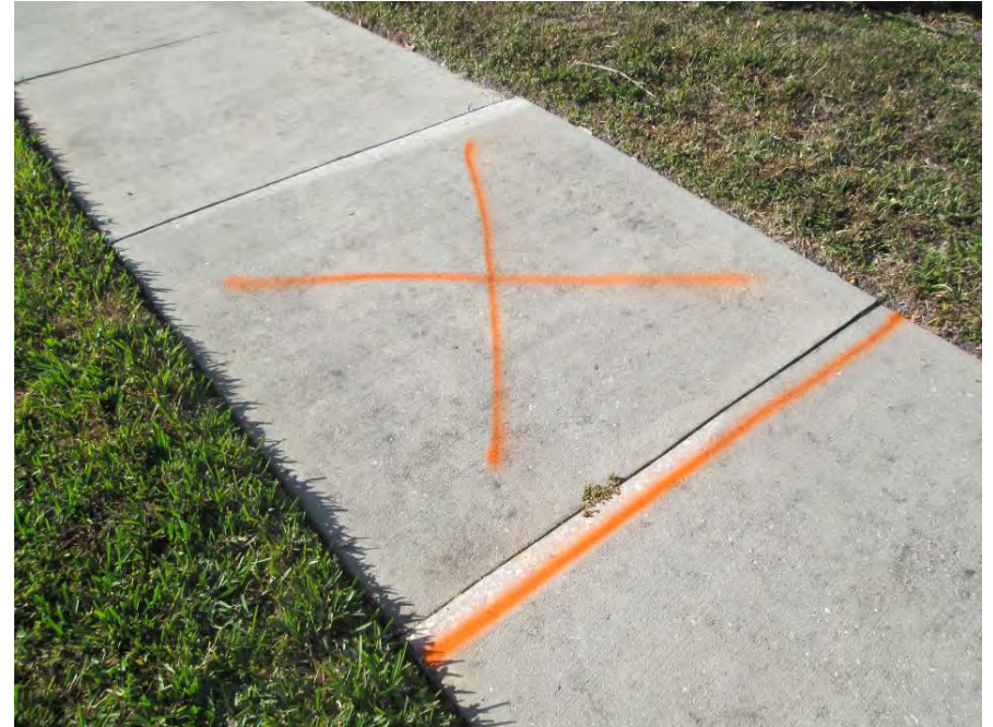
Remove & Replace 5.5' x 5' on east end of Brookfield Terrace
