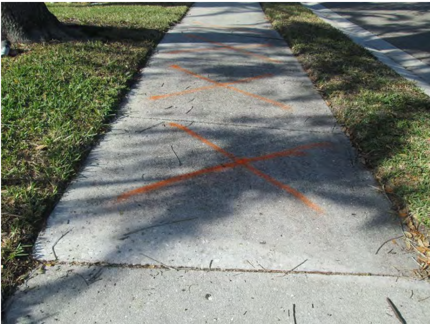
Remove & Replace 20' x 5' on Heritage Isles Way at Fairway Isles Lane
