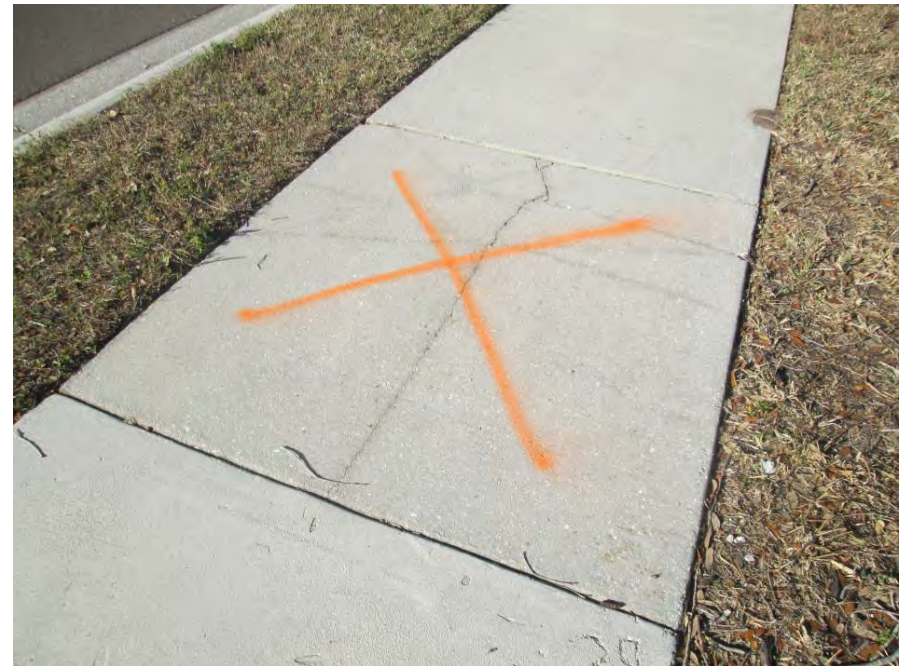
Remove & Replace 5' x 5' on south end of Golden Harbour Dr
