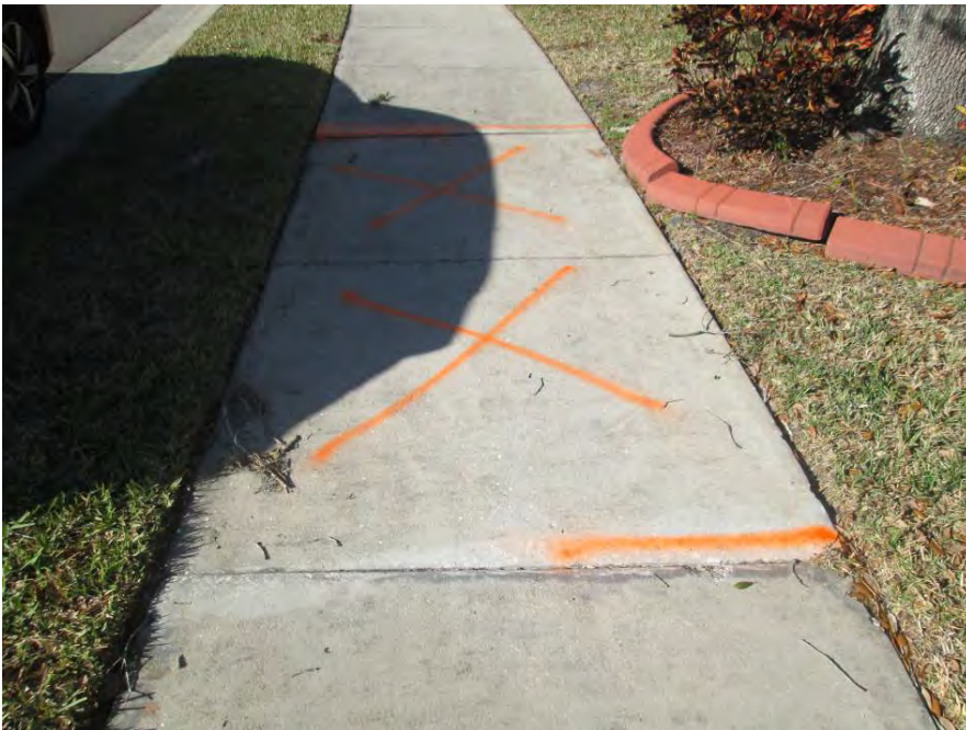
Remove & Replace 10.5' x 5' on Brookfield Terrace
