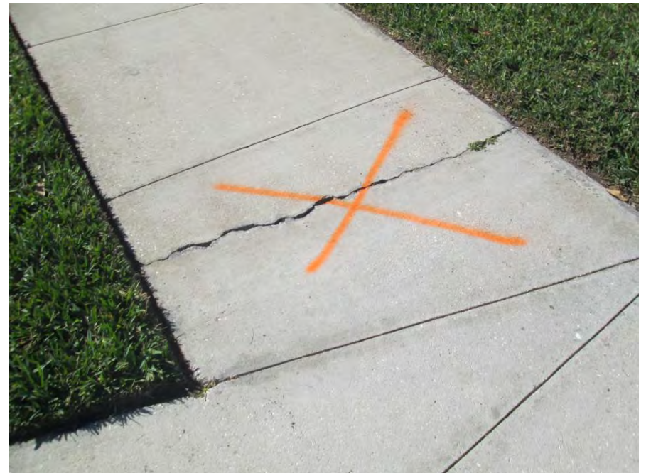
Remove & Replace 3.5' x 5' on Summer Green Terrace
