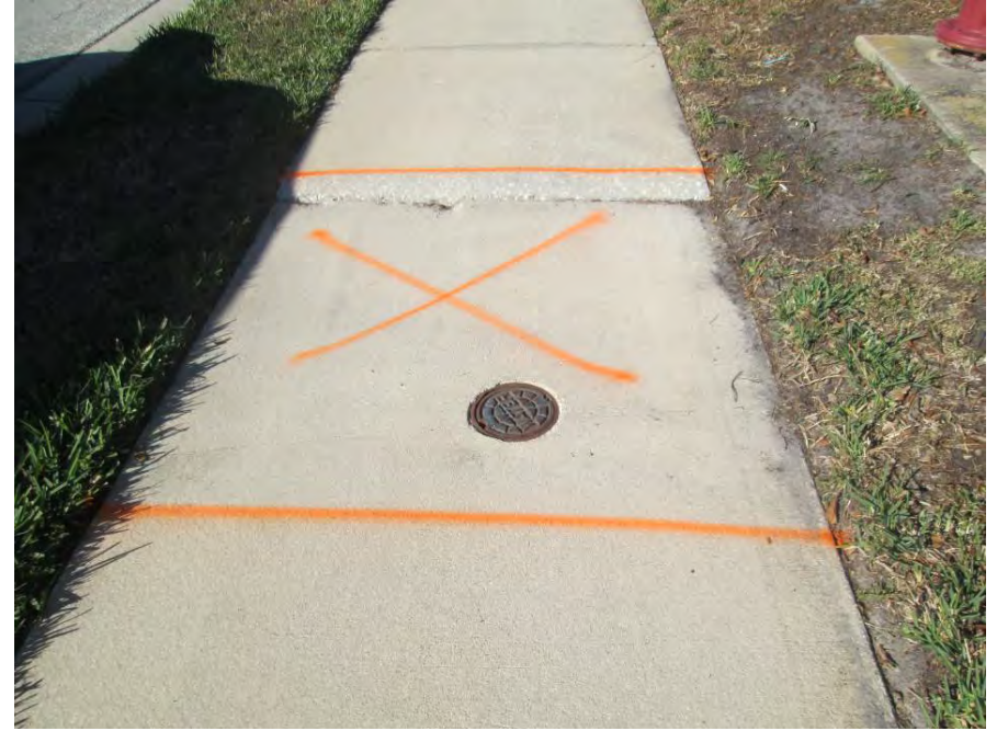
Remove & Replace 5.5' x 5' on west Stone Harbour Loop, adjust valve cap
