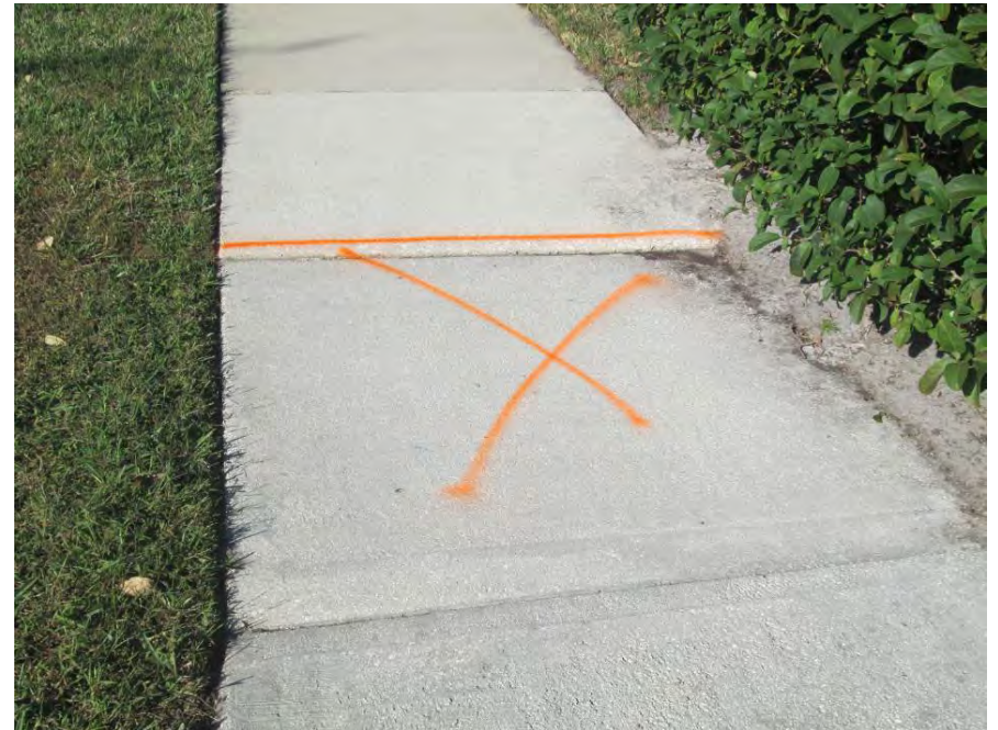
Remove & Replace 5.5' x 5' on west Stone Harbour Loop
