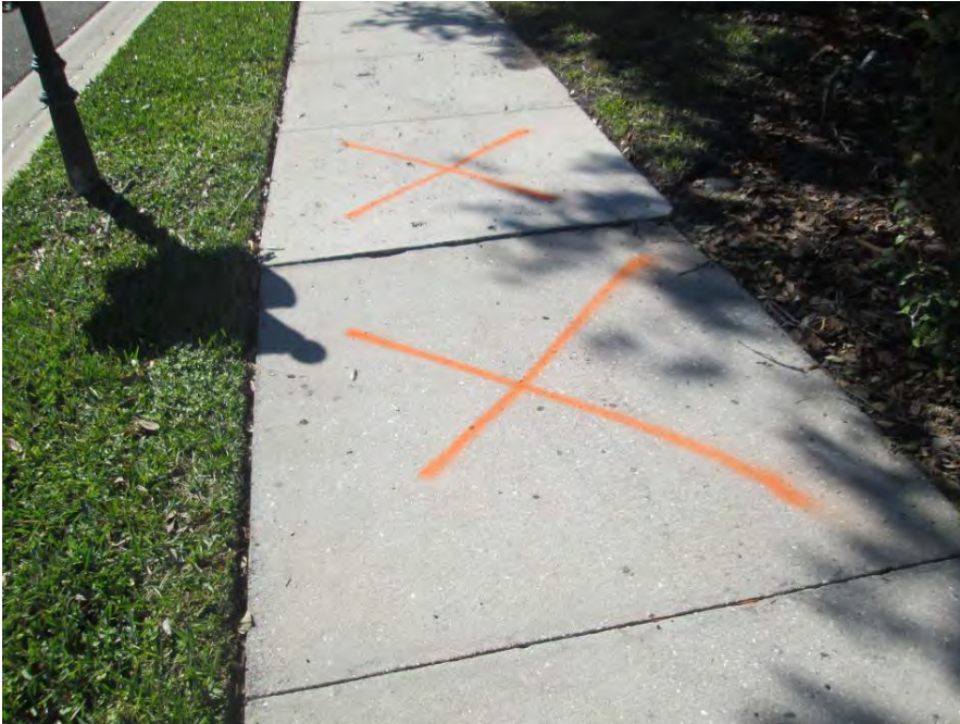
Remove & Replace 10' x 5' on Summer Green Terrace
