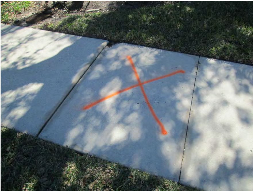
Remove & Replace 4' x 5' on west Montauk Point Crossing
