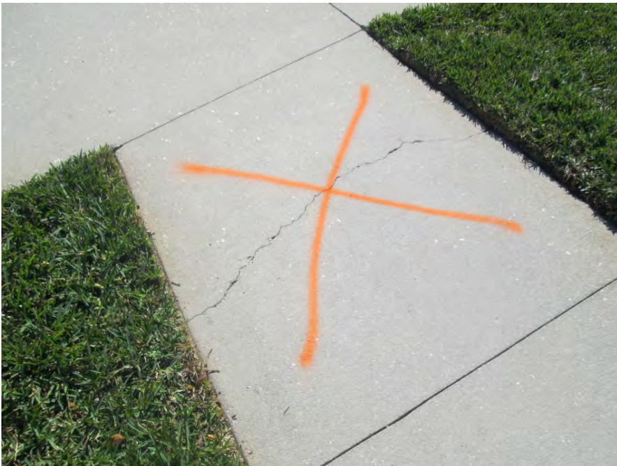
Remove & Replace 6' x 5' on Monterey Bay Loop
