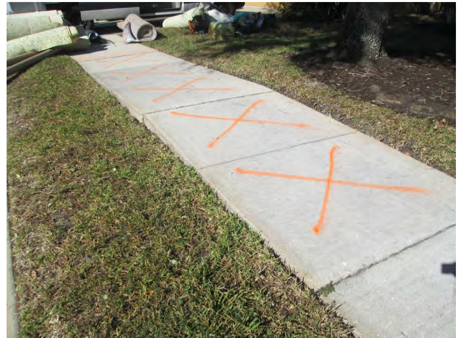
Remove & Replace 21' x 5' on east Stone Harbour Loop s/o Heritage Inlet Pl
