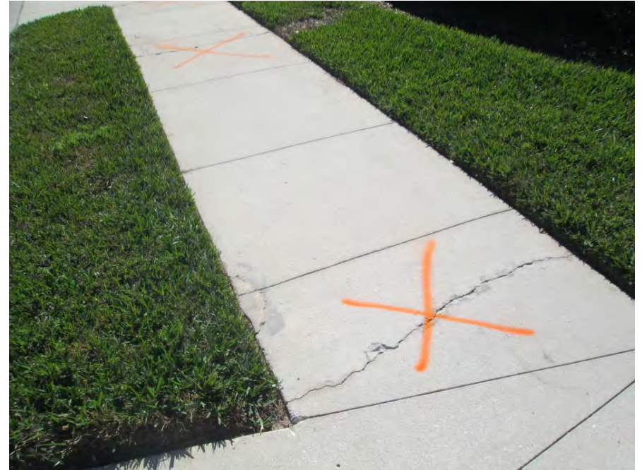
Remove & Replace 3'x5', 5'x5' & 3.5'x5' on west Stone Harbour Loop
