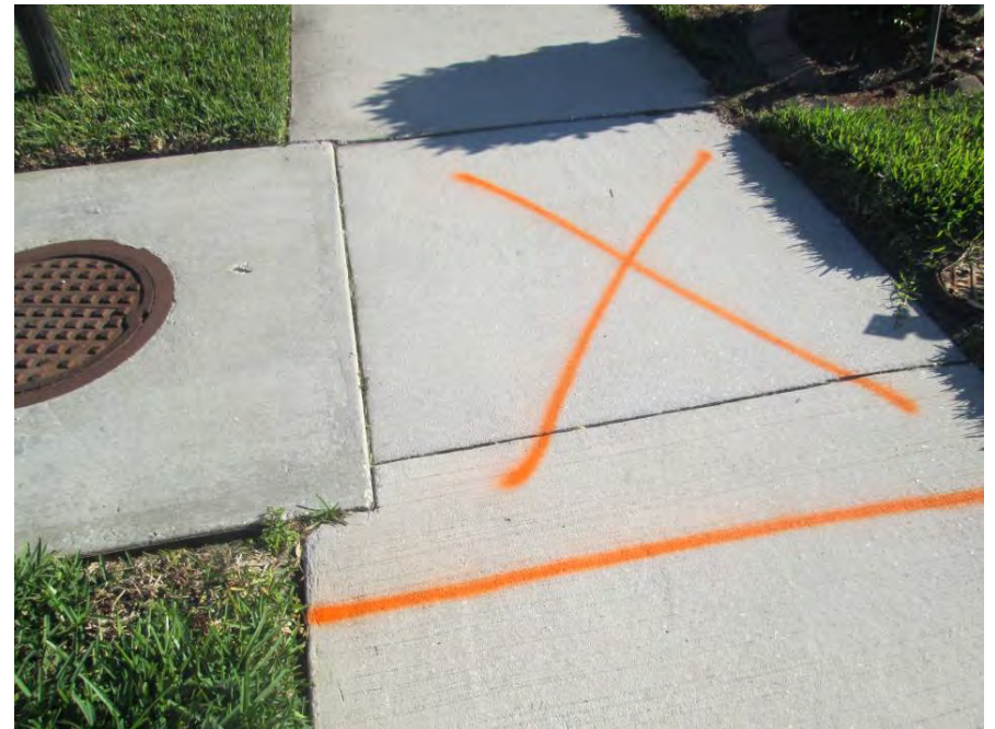
Remove & Replace 6'x 5' on east Camden Harbour Loop n/o Haven Harbour
