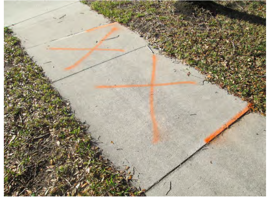
Remove & Replace 9' x 5' on Kinsbury Place
