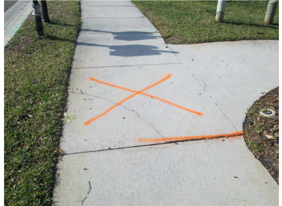
Remove & Replace 5'x5' on Camden Harbour Loop near Heritage Isles Way
